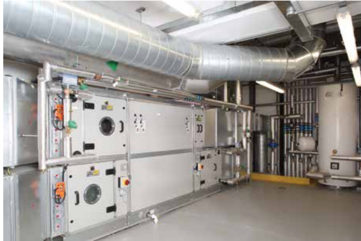
Functional plant room, demonstrating a considered and logical approach
