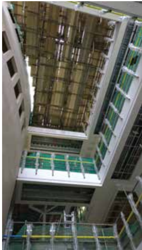
BDH Atrium during construction.
