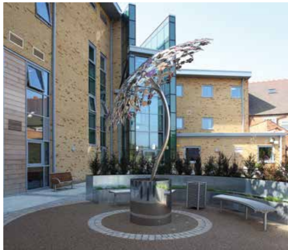
Roof garden courtyard with car park beneath
