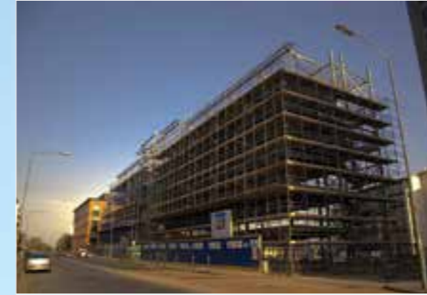
Inset: During construction
